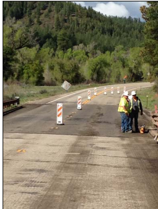
Sawcutting asphalt curb
