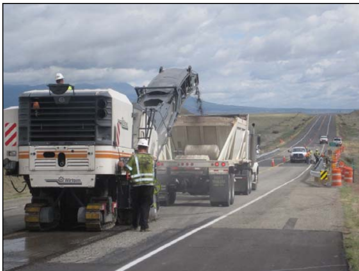
Milling northbound lane at Indian Creek
