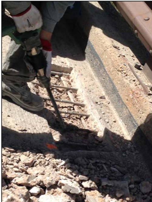
Class II Bridge Deck Repair
